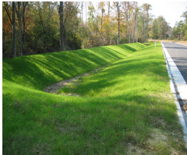
Swale provides temporary storage for storm water & reduces peak flows.
