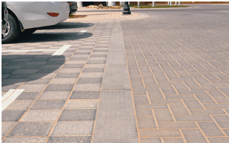
Flush Slipform Concrete Kerb
