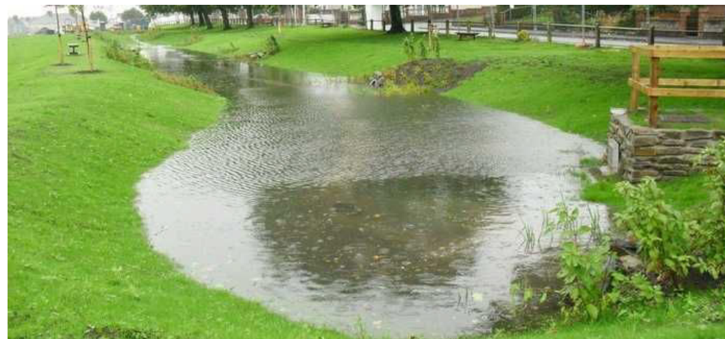
Typical swale in wet weather
