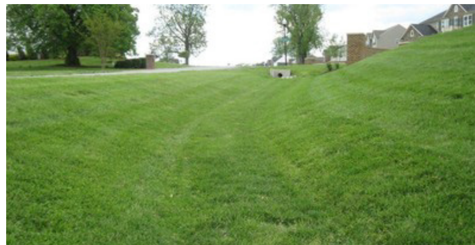
Typical swale in dry weather
